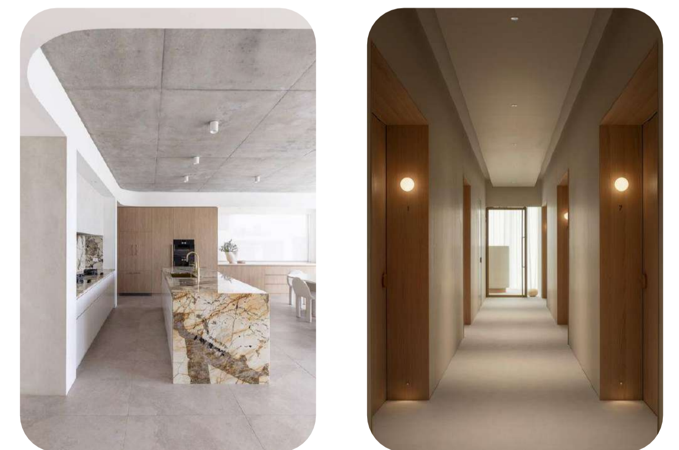
EXPOSED CONCRETE CEILING WITH PLASTERBOARD BULKHEADS AND CEILINGS OVER CORRIDORS AND BATHROOMS
