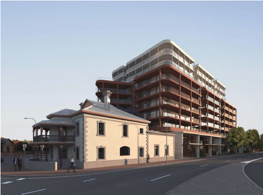
Figure 15 – View north from pedestrian median on Walkerville Terrace
